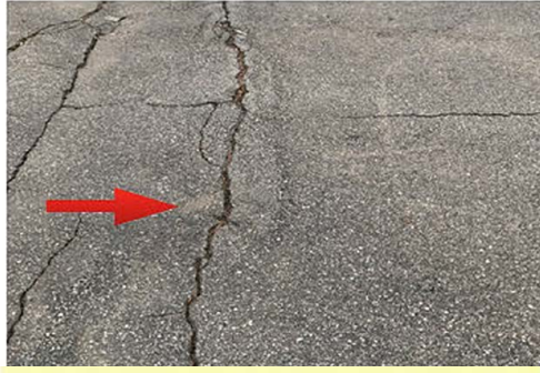
Example of damaged concrete.
