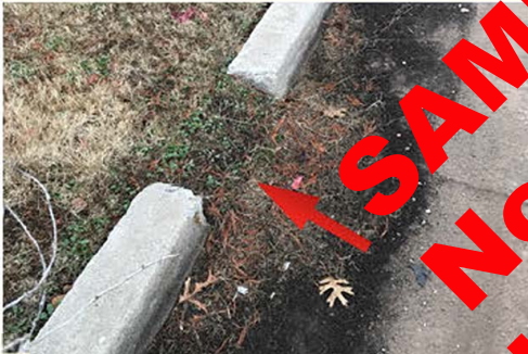
Example of improper landscaping
